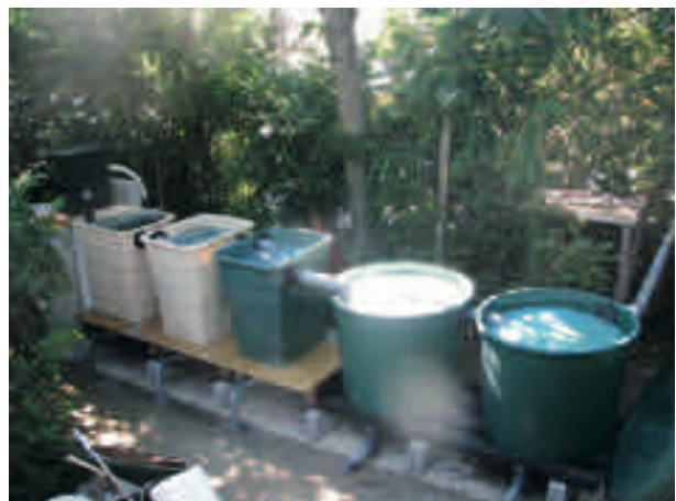
Above: Filtration systems using biomedica, made from garden waste bins © D.R.
