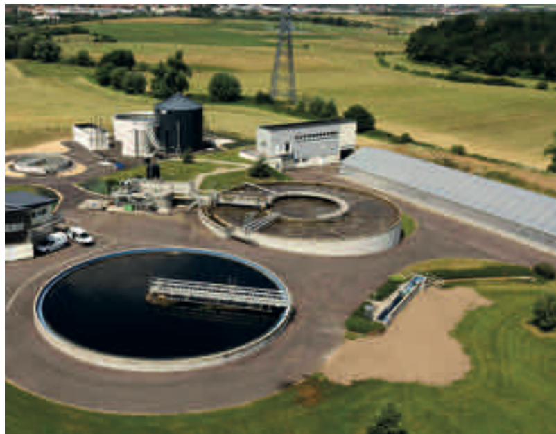
Below: Wastewater treatment plant in the town of Folschviller © All rights reserved
