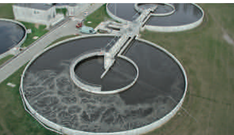
Above: Activated sludge plant © IRSTEA
