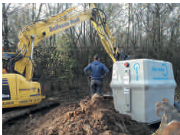
Above: Installation of a micro purification Oxyfix® plant ©Eloy Water ( www.elaywater.fr )
