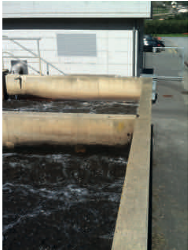
Above: Uncovered bioreactors at Saillon in Switzerland were the source of the biomedica lost to the environment © Surfrider Léman
